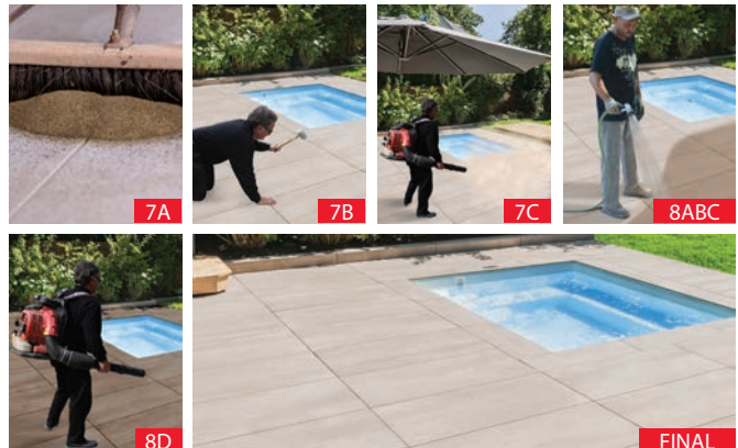
GATOR TILE SAND INSTALLATION STEPS
